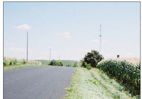
WisDOT Tower on Maple Road
